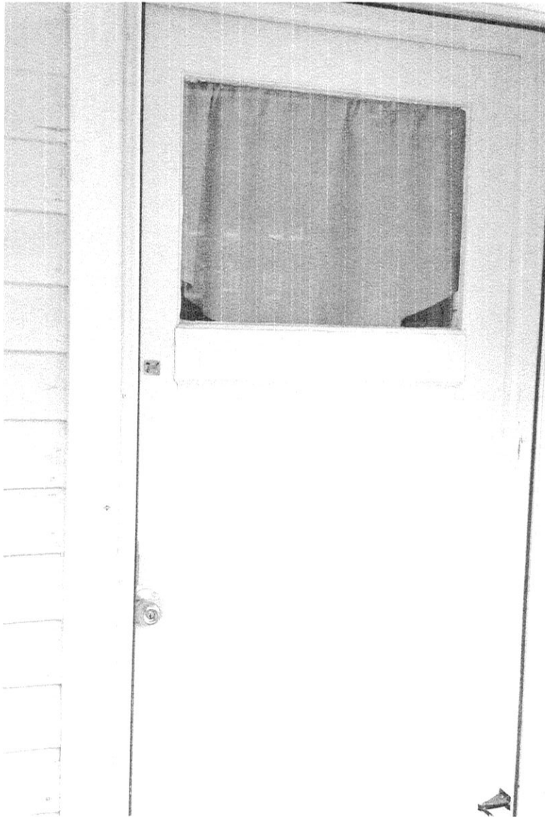
2nd floor door
