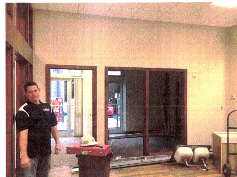
North partition to be removed
