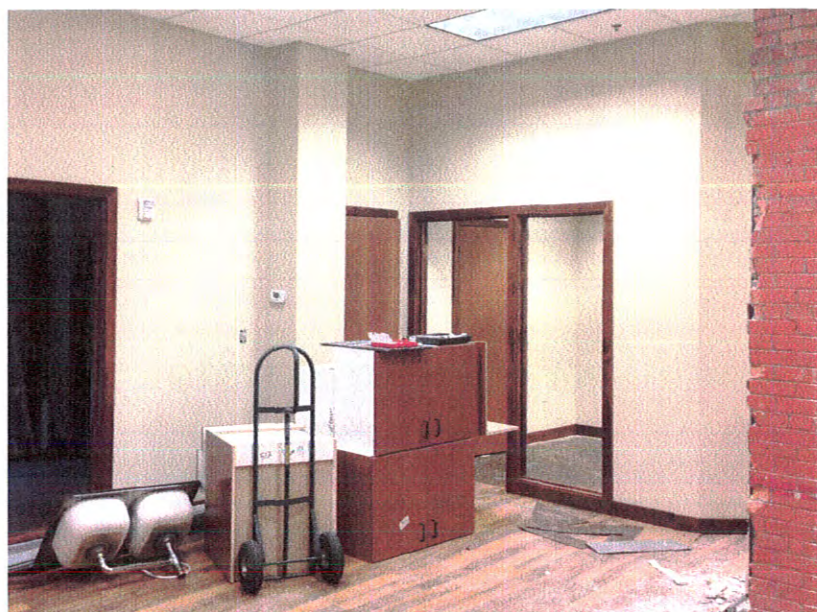
East wall to be removed
