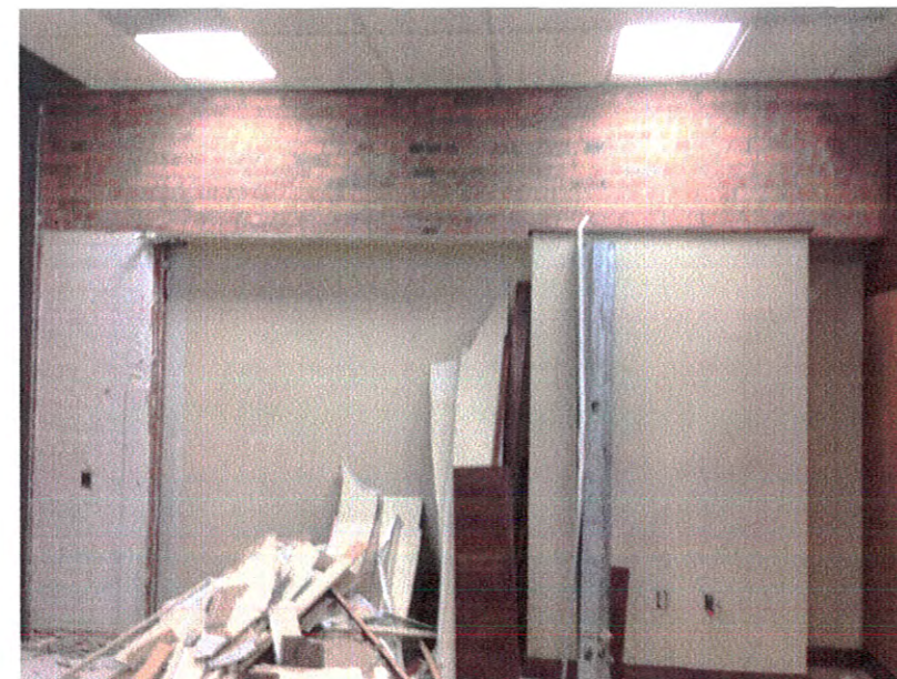
South brick wall exposed
