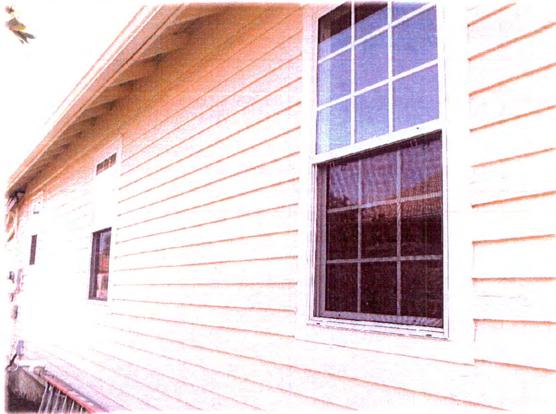
Windows on the north side of the house.
