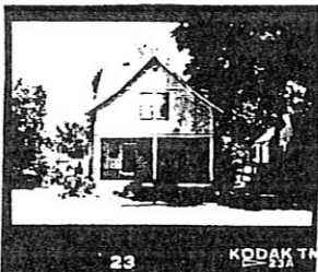
Two-story gable-fronted house with wood shingles in upper gables and double hung windows.
