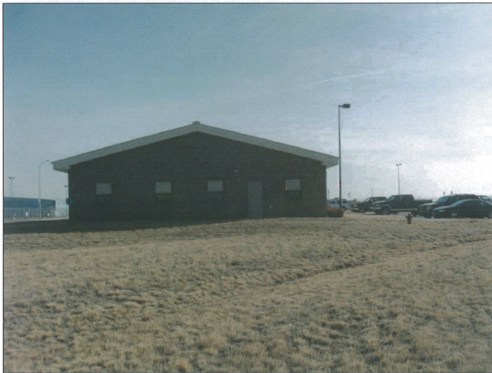
Photograph 6 – View of northeastern adjacent property.
