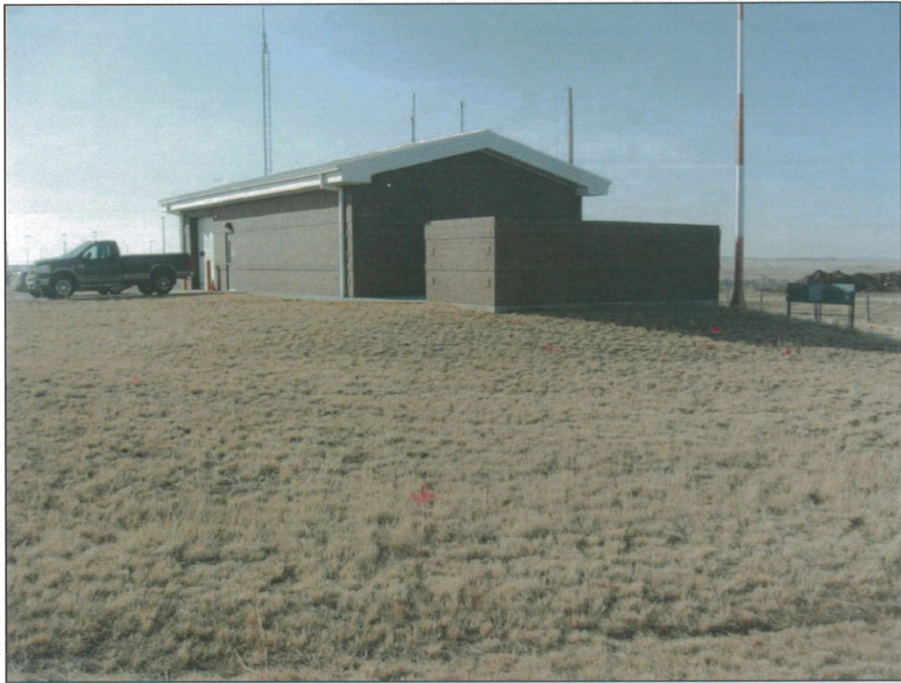
Photograph 3 – View of subject property facing south.
