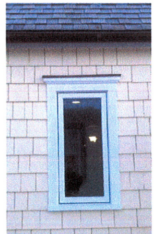
Kitchen window – replaced 2009. Note trim and compare to original.
