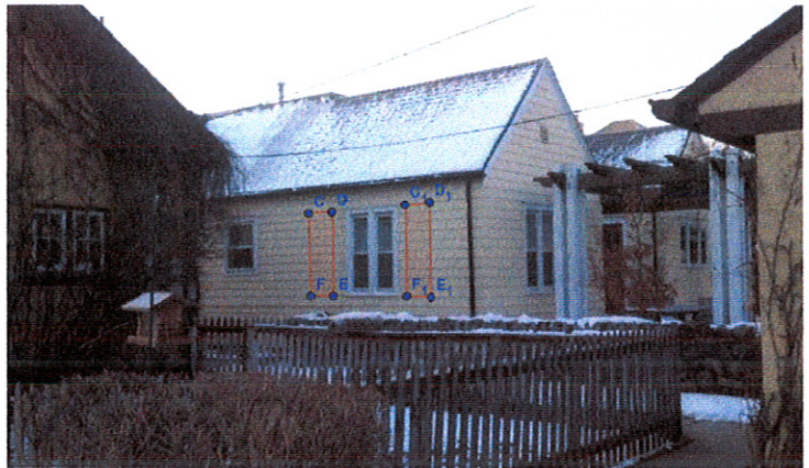
View of north side of house looking south east from St. Cloud St. Note locations of proposed windows.
