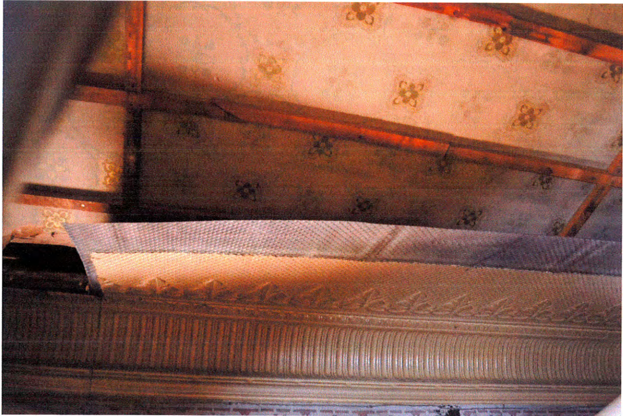
ceiling wall paper, stenciling, + molding left intact, + exposed
