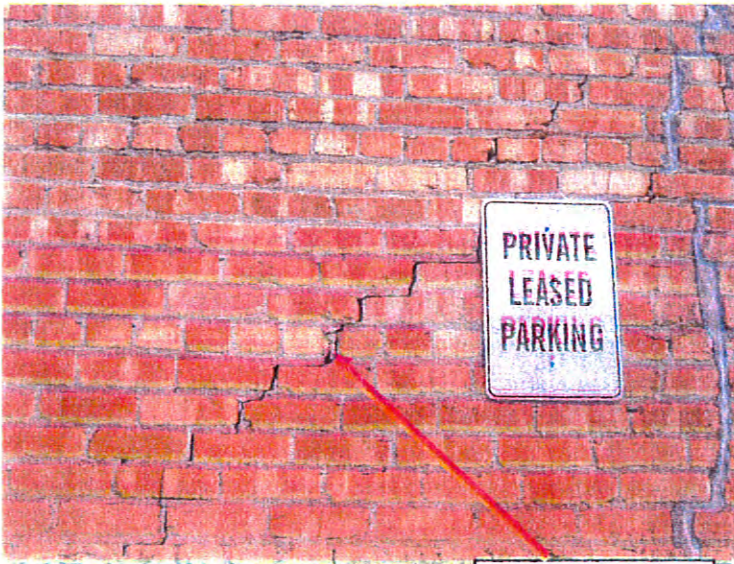
Typical settlement cracks to be resealed
