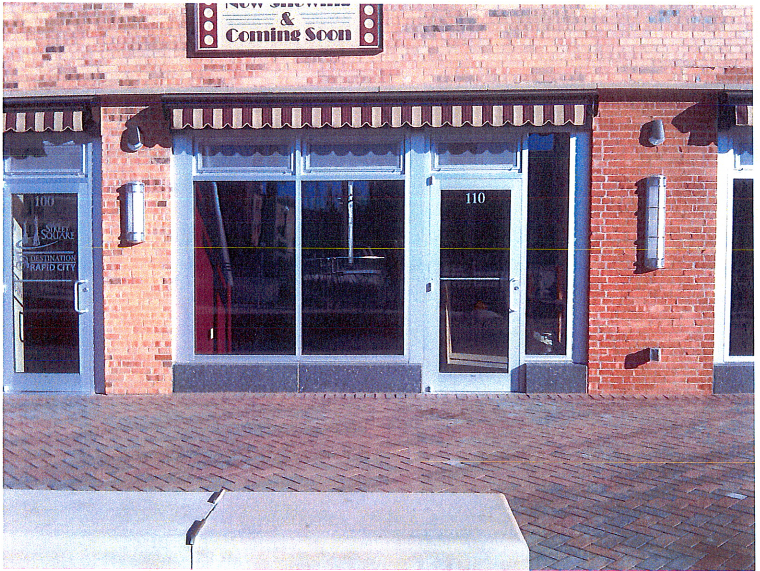
Exterior view of pass three window location
