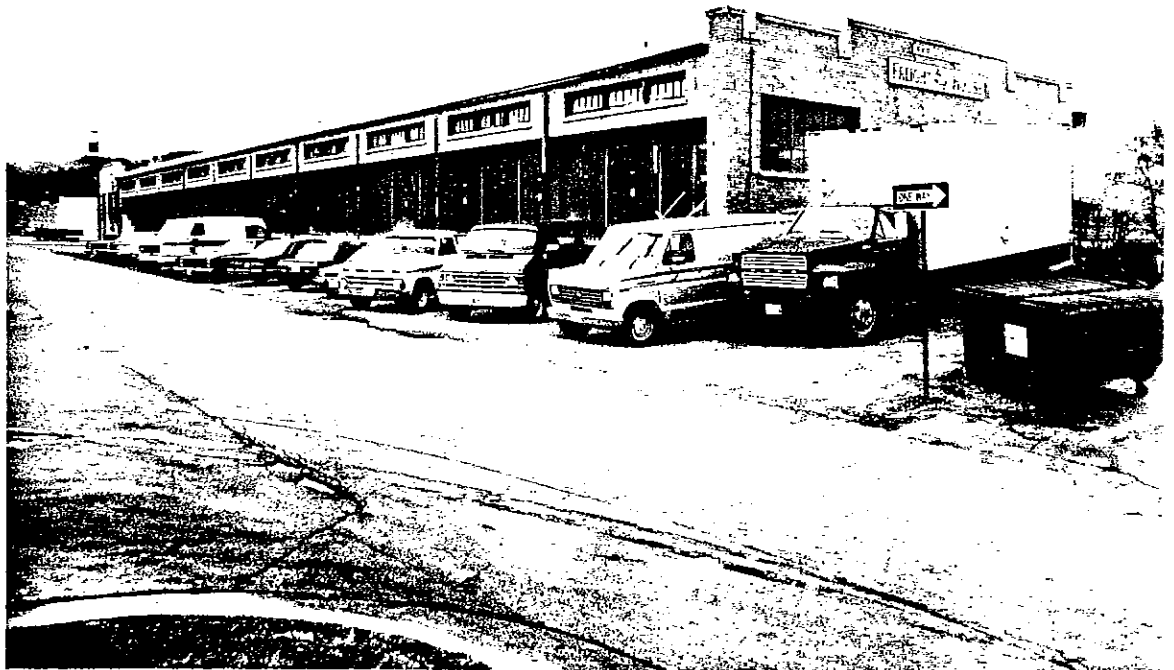
Milwaukee Road Freight House, Pennington County, S. Dak., No. 4
