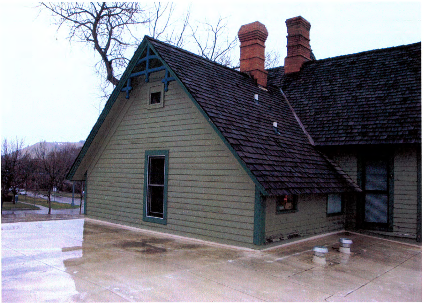
⑧ SOUTH ELEVATION, SECOND FLOOR, ON ROOF
