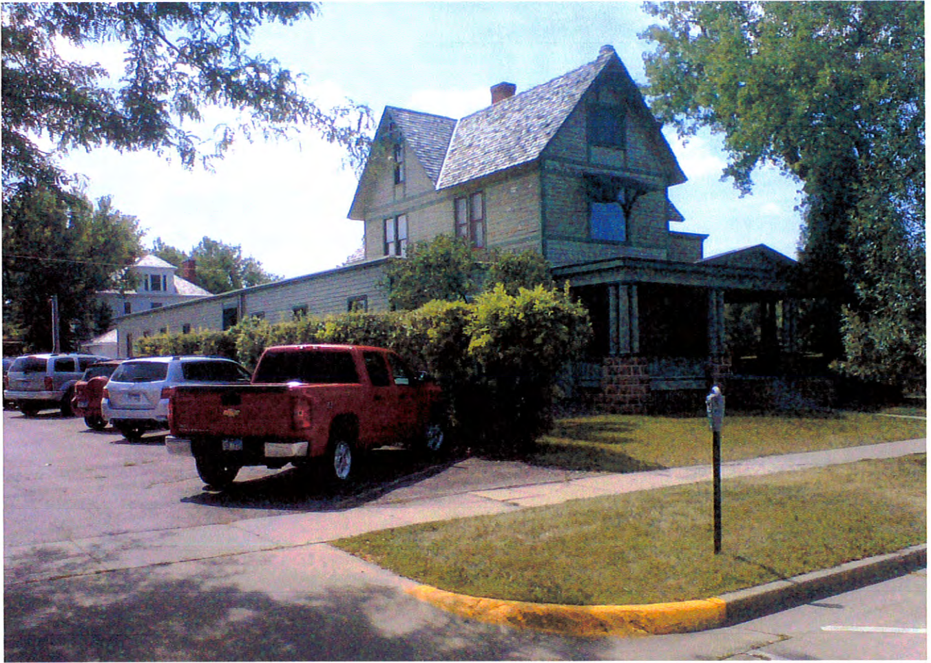
⑥ NORTHEAST CORNER
