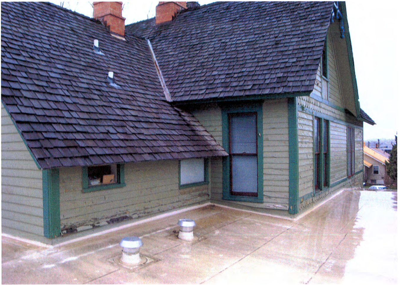
⑨ EAST ELEVATION, SECOND FLOOR, ON ROOF
