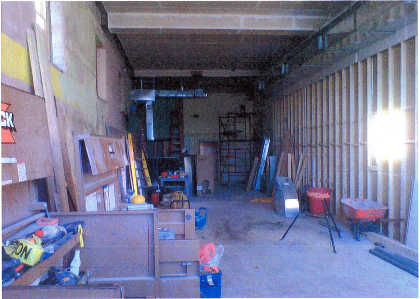
⑤ INTERIOR VIEW LOOKING SOUTH
