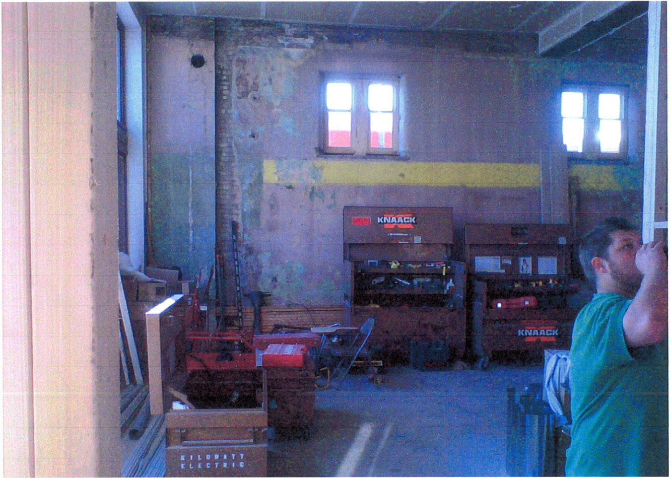
④ INTERIOR VIEW LOOKING EAST
