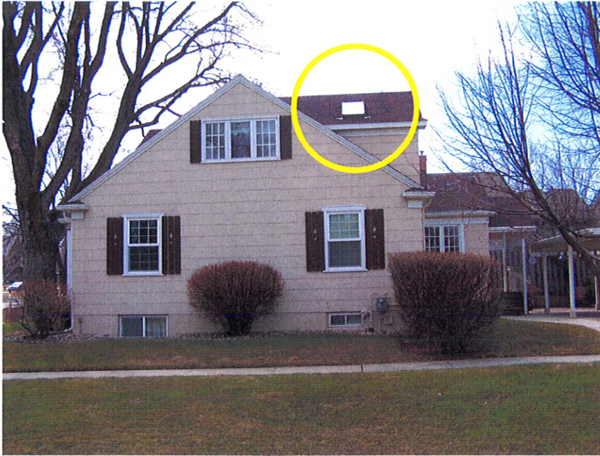
Side View of Home - taken from Franklin Street
