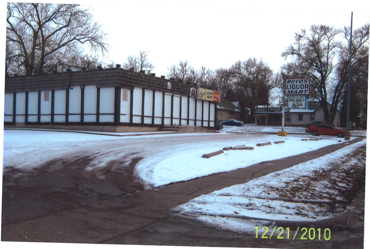
West side of existing building – looking south
