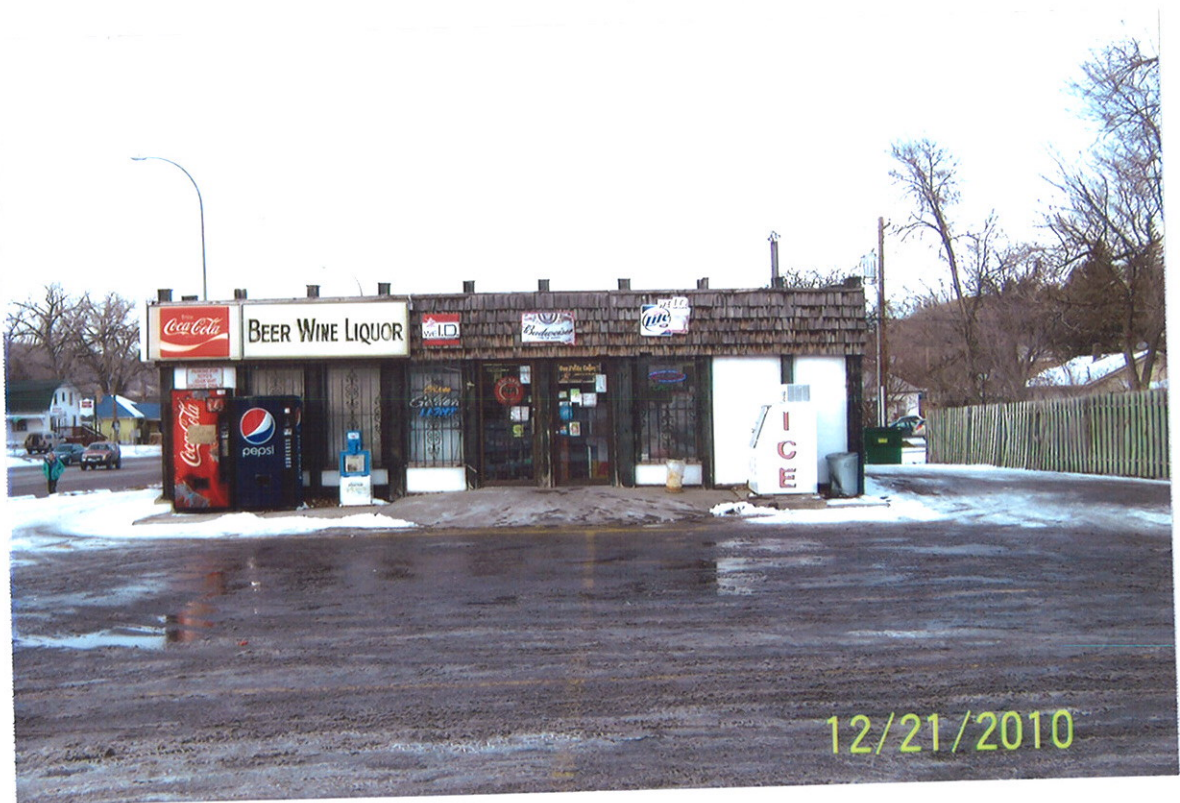
South face of existing building
