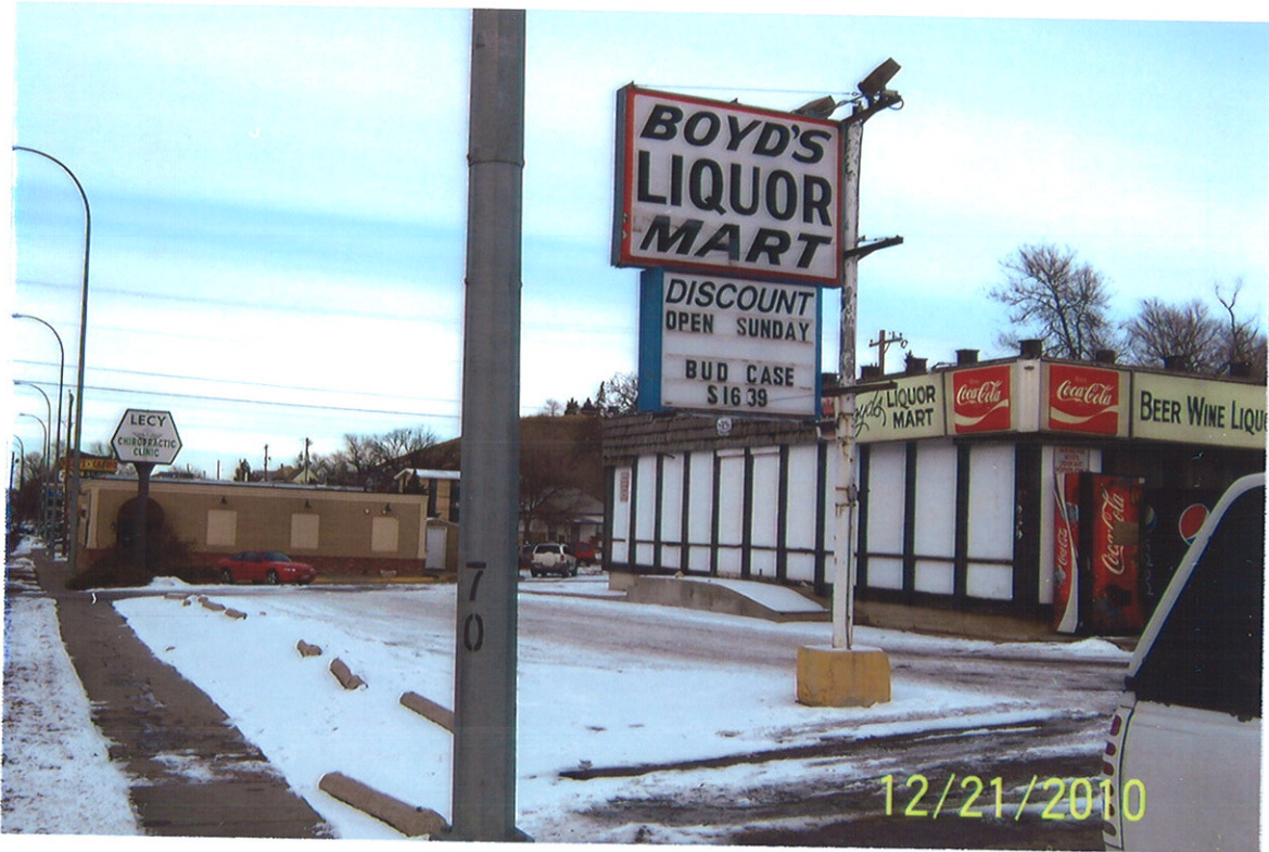
West side of existing building – looking north
