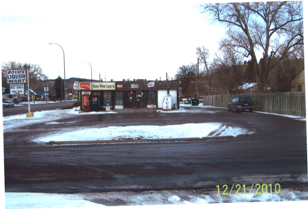
South face of existing building – from across St. Cloud Street
