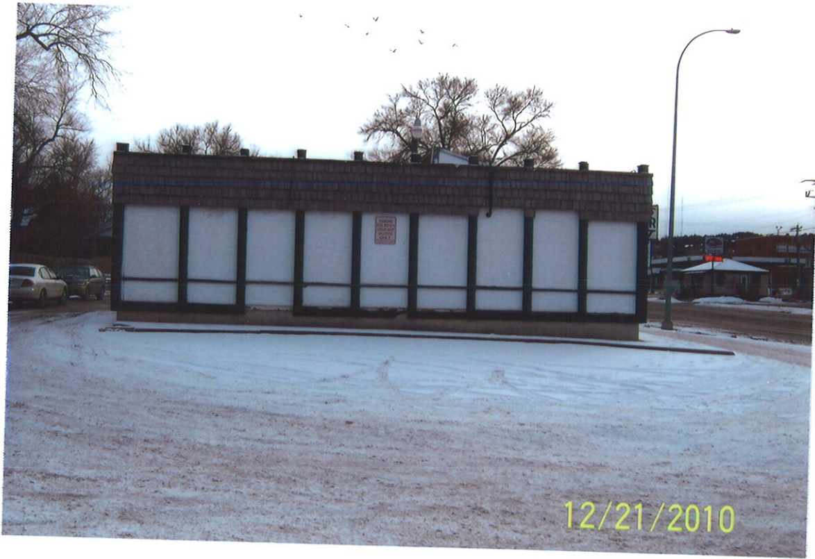
North face of existing building
