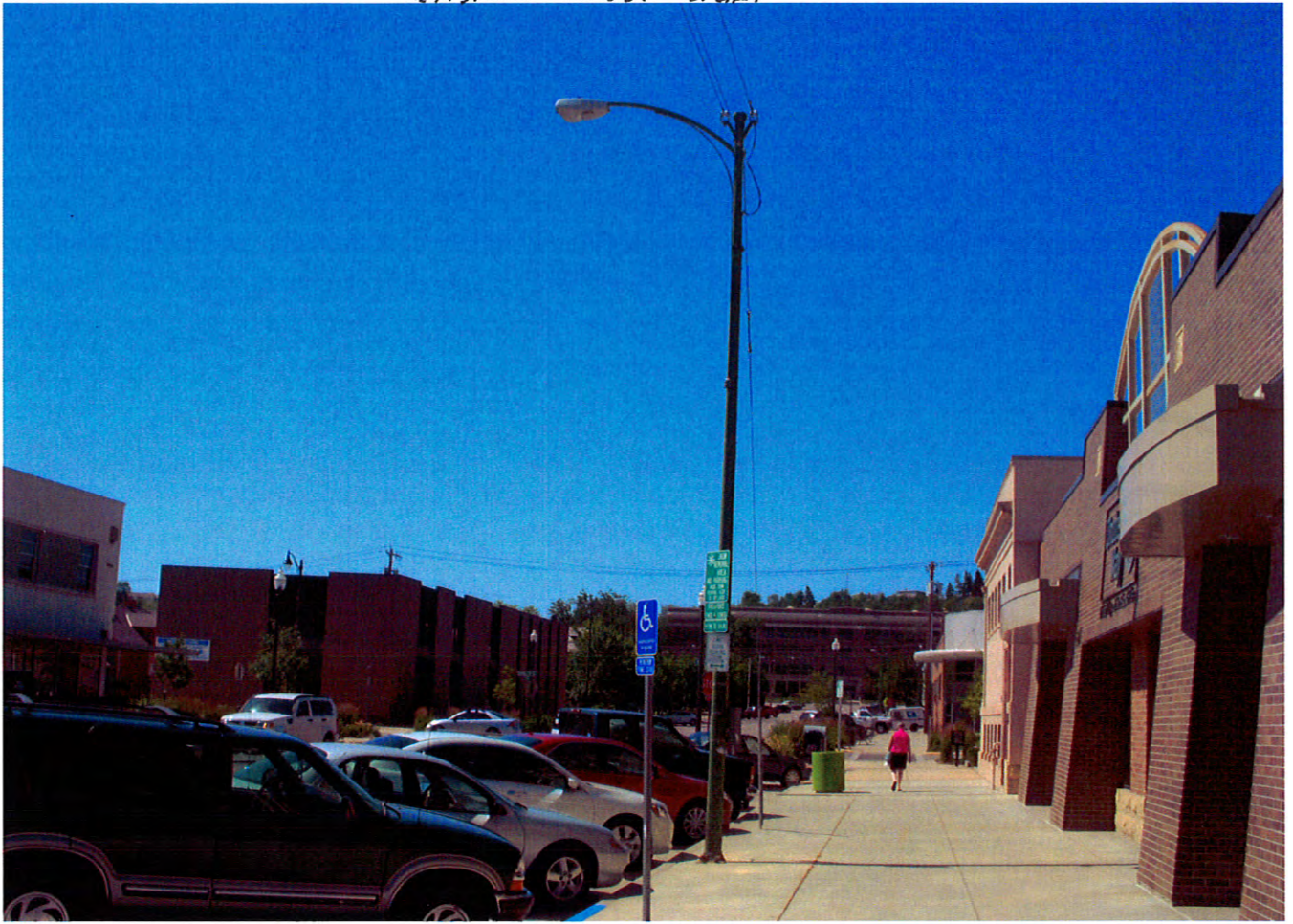
EXISTING STREET LIGHT
