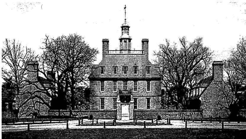
In the 1930s reconstruction of the 18th century Governor's Palace at Colonial Williamsburg, Virginia, the earliest archeological remains of the brick foundation were carefully preserved in situ, and serve as a base for the reconstructed walls. Photo: The Colonial Williamsburg Foundation.
