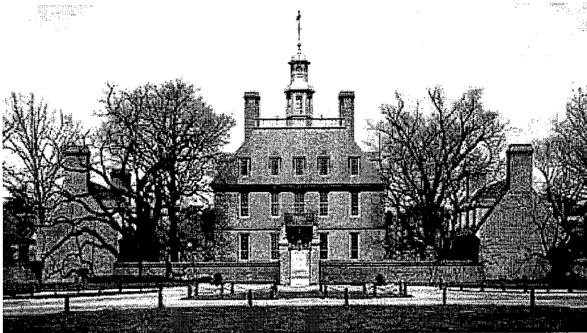
In the 1930s reconstruction of the 18th century Governor's Palace at Colonial Williamsburg, Virginia, the earliest archeological remains of the brick foundation were carefully preserved in situ, and serve as a base for the reconstructed walls. Photo: The Colonial Williamsburg Foundation.
