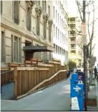
The ramp's scale and materials are inconsistent with the historic character of the building. Photo: NPS files.
