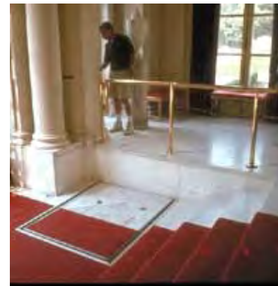
A retractable lift for this historic building foyer was created using "like" materials. Photo: NPS files.
