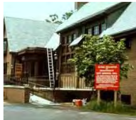
This accessibility ramp is compatible with the historic building in scale and materials. Photo: William Smith.
