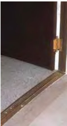
The historic threshold was made accessible with a 1/2" wood bevel.
