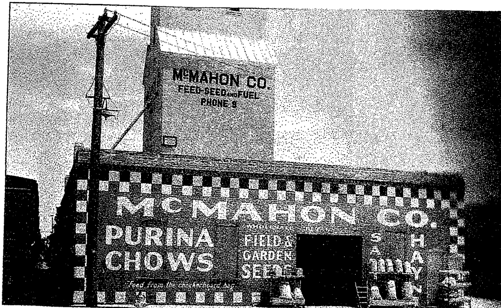
The McMahon Company, founded in 1896, served the needs of the area's agricultural and farming community. Expanding to six buildings by the railroad tracks, a grain elevator was added in 1911. The T. E. Ibberson Company of Minneapolis built the elevator, which has a gable roof and corrugated metal siding. The first structure was a single-story brick flat-roofed building with a roofline dentil course and eyebrows over openings providing minimal decoration.
