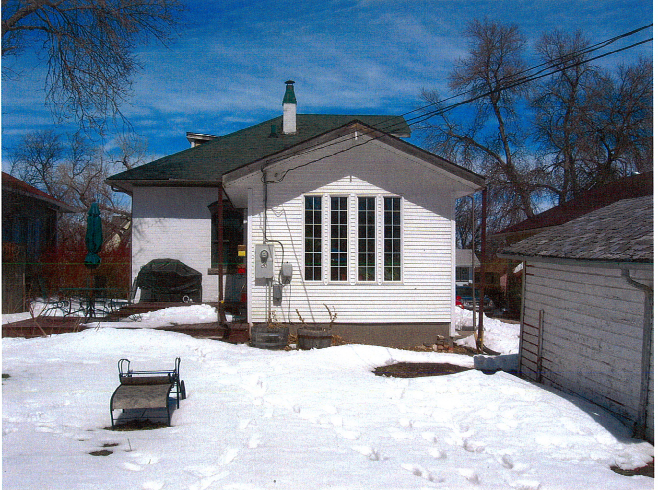
Photo 3 – House from rear – taken from the center of the lot. The sunroom addition was added in 1995. It has vinyl siding and a 4/12 roof pitch
