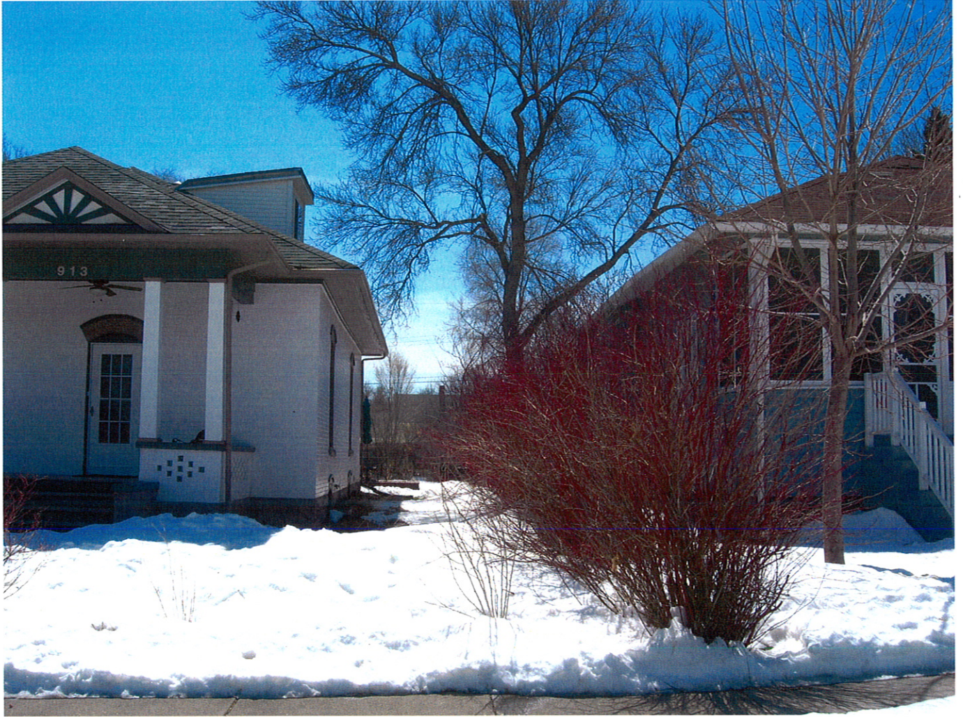
Photo 2- Front from side walk showing the west side view
