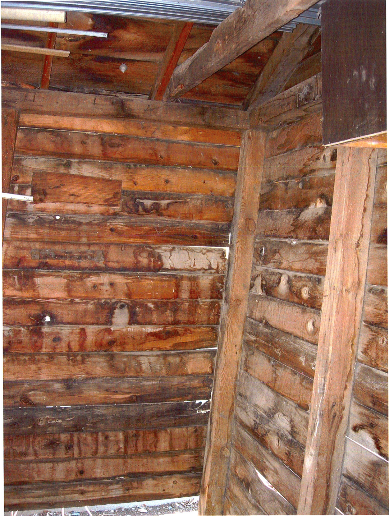
Photo 1 – interior southeast corner
