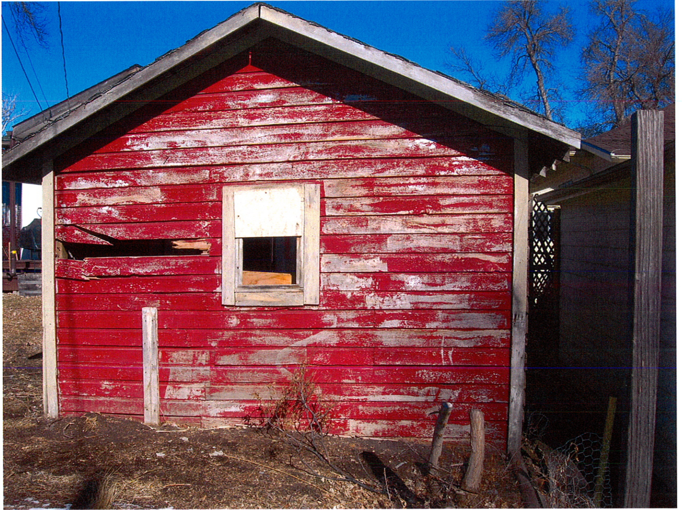
Photo 4 – Shed exterior south wall
