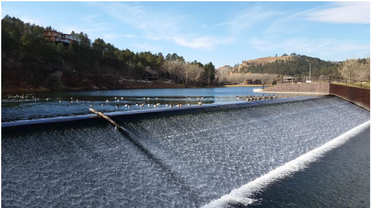
Photo 4. Canyon Lake Dam Reconstruction
