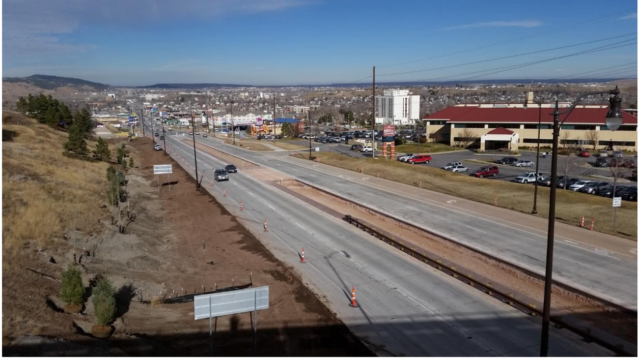
Photo 5. Mt. Rushmore Road Corridor Project
