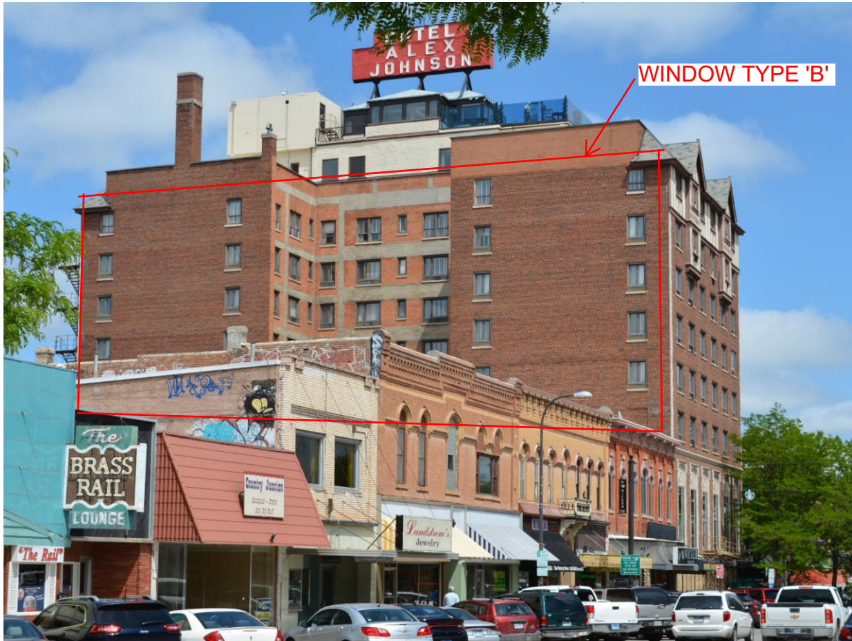
WEST SIDE OF BUILDING
