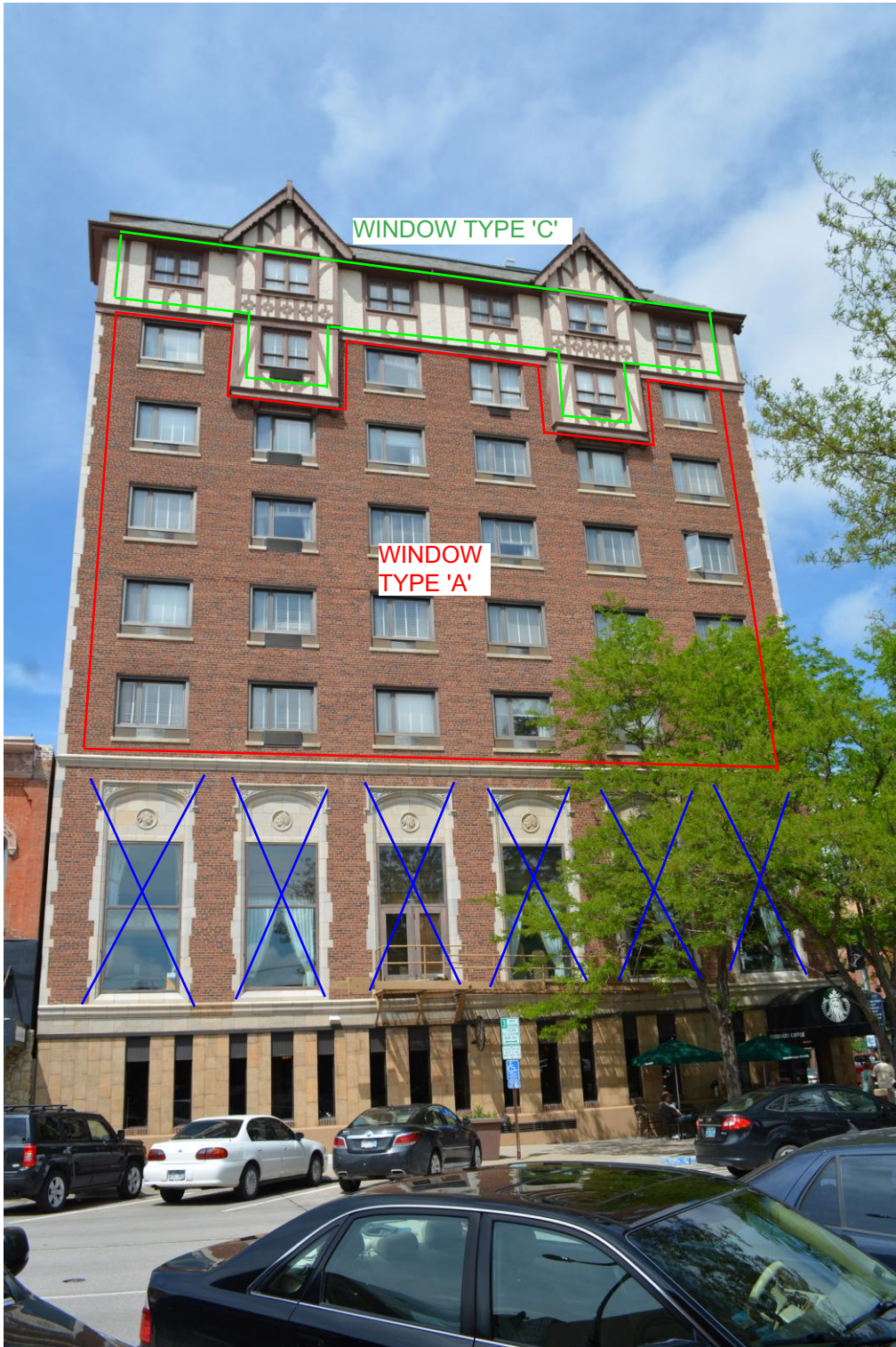
SOUTH SIDE OF BUILDING
