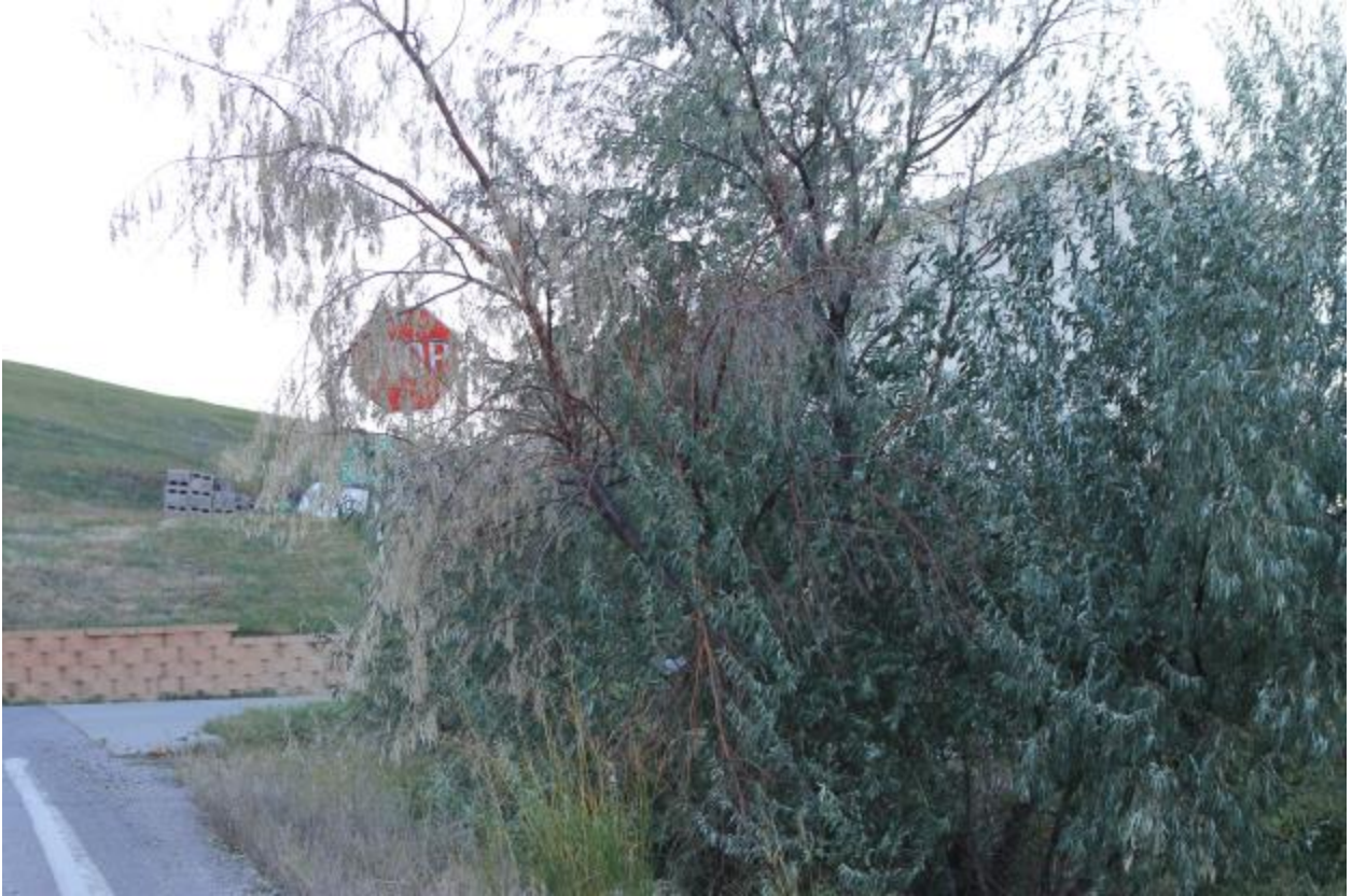
Tree blocking stop sign.
