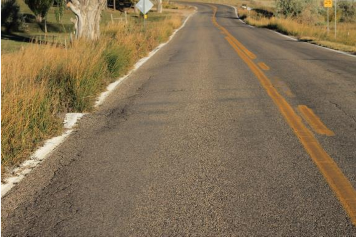
Culvert with a dip all the way across
