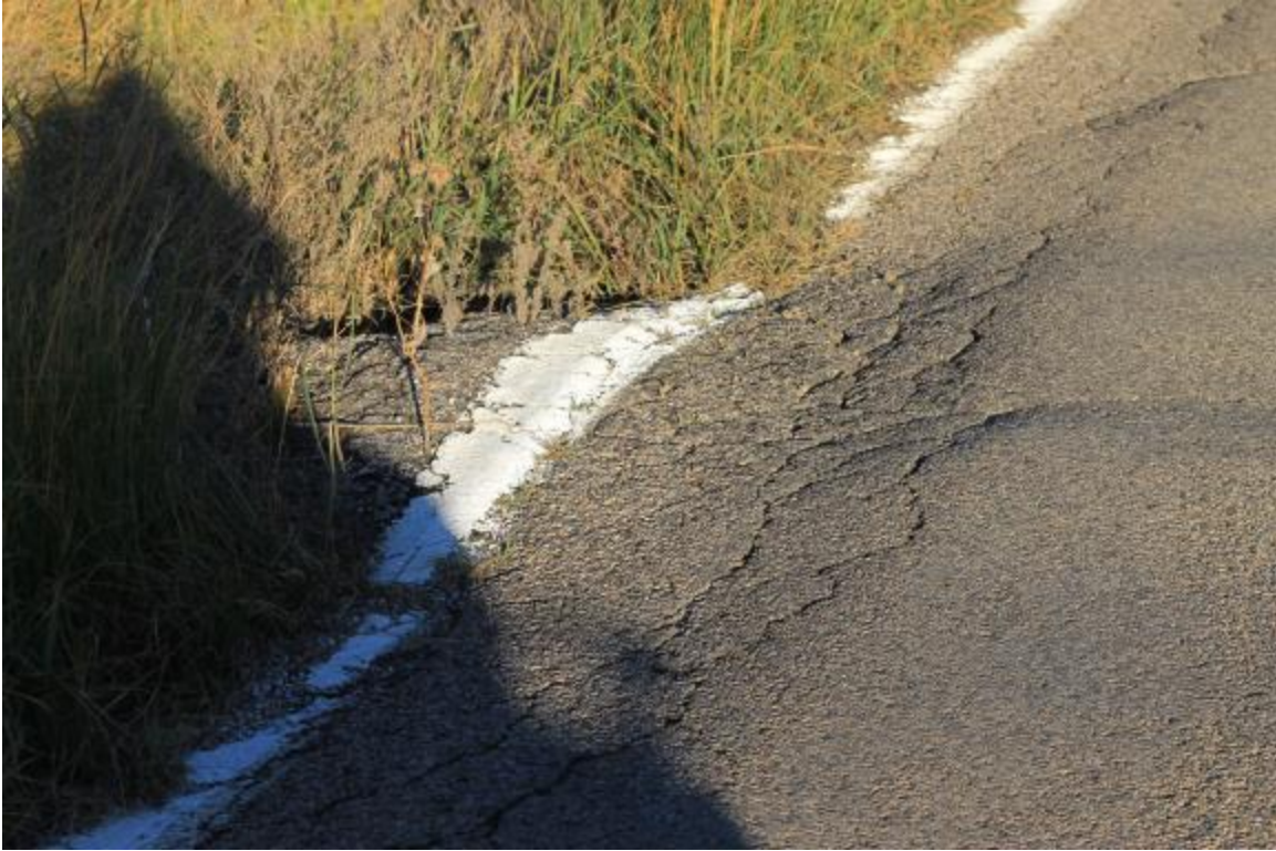
Culvert opposite a patch.
