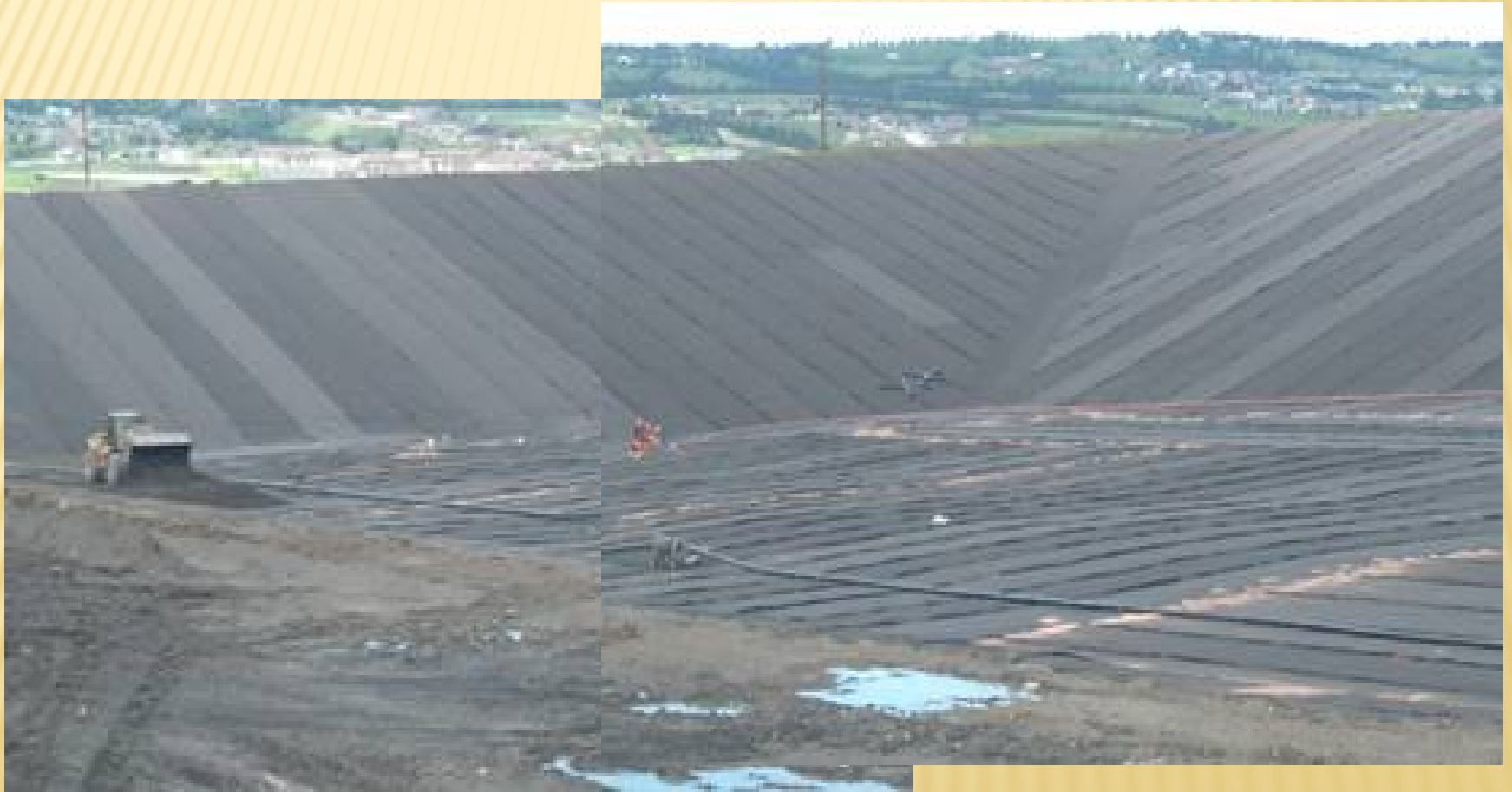
Cell 16 Liner Construction
