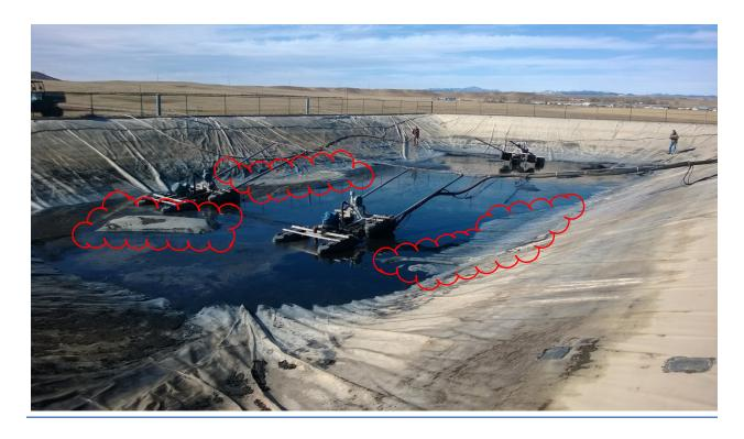
March 14, 2014 photo of the 750,000 gallon sludge pond cell. Highlighted areas indicate locations where the liner is visibly floating.
