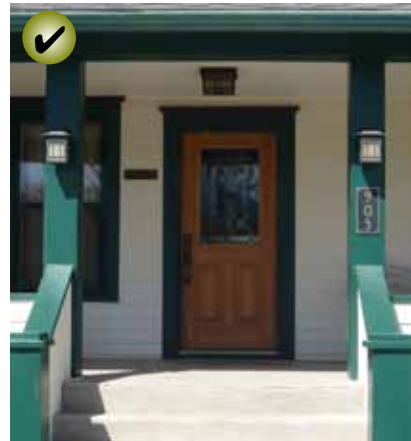
When replacing a door, use materials that appear similar to that of the original.
