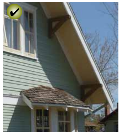
Protect wood features from deterioration.
