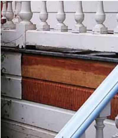
Repair deteriorated building materials by patching, piecing-in, consolidating or otherwise reinforcing the material.
