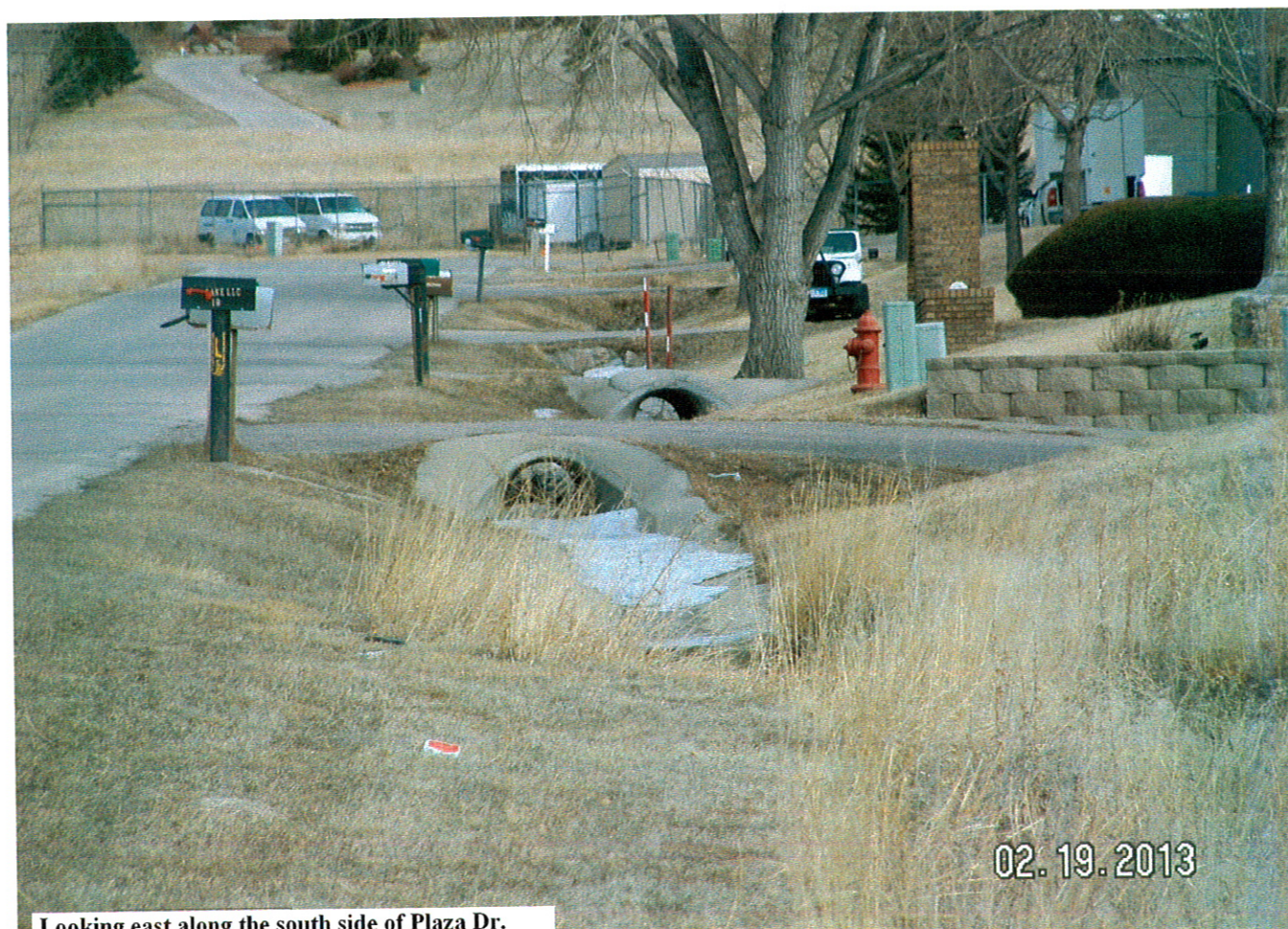
Looking east along the south side of Plaza Dr.
