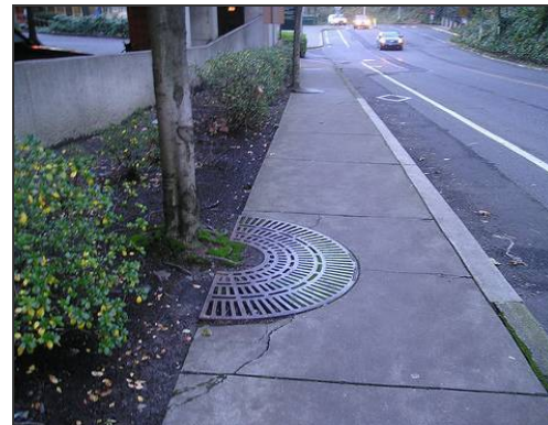
Tree well grates can create uneven sidewalk conditions and should not be placed within the thru-pedestrian zone.
