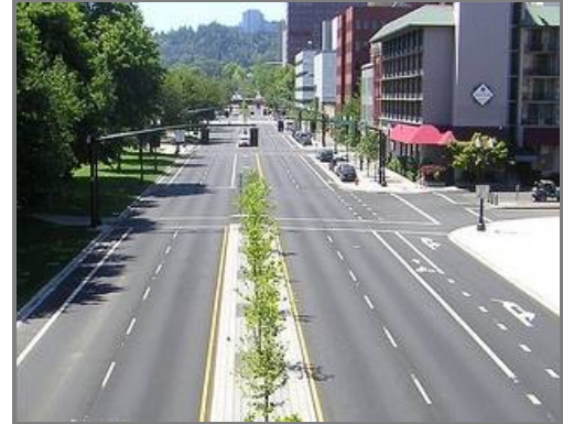
This street previously had 13' lanes, which were narrowed to accommodate bike lanes without removing a lane.
