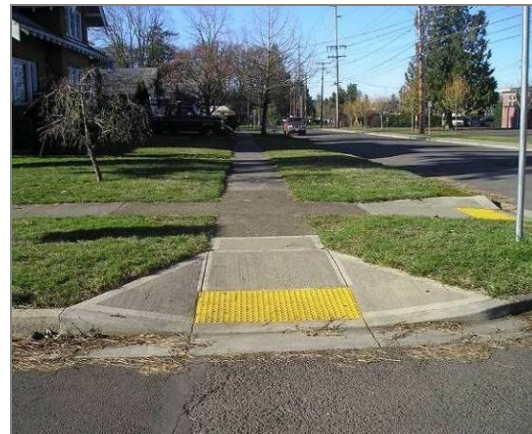
Example of an ADA-compliant perpendicular curb ramp
