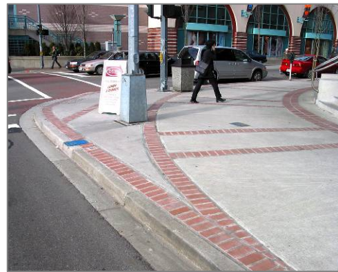
Figure 59. Reducing the radius of a turn reduces traffic speed and greatly improves safety for bicyclists and pedestrians
