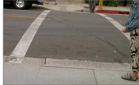
Parallel markings are the most basic crosswalk marking type, and are applied where textured concrete crosswalks are used.
