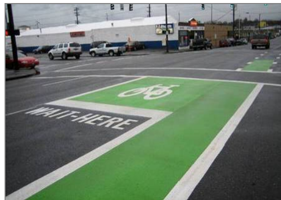
Bike boxes have been installed at several intersections in Portland, OR where right-turning motorists conflict with through bicyclists
