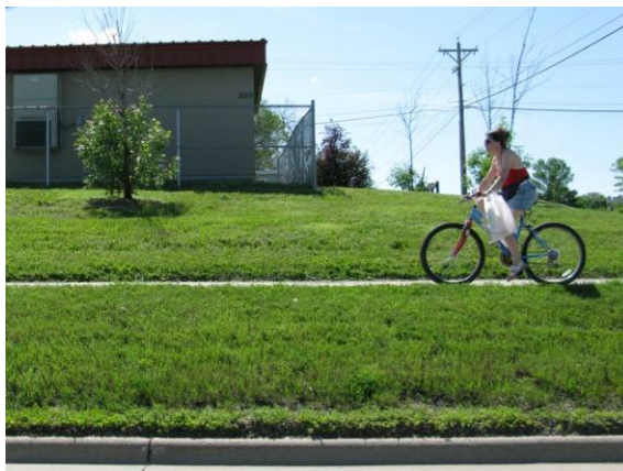
Example of a substandard side path
