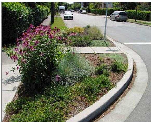
Figure 41. Planted curb extension in Portland, OR
