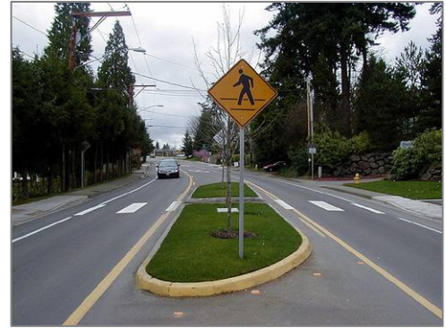
Figure 42. Pedestrian refuge island at mid-block crossing.
