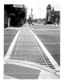
Raised crosswalks are Speed Tables outfitted with crosswalk markings and signage to channelize pedestrian crossings, providing pedestrians with a level street crossing. Also, by raising the level of the crossing, pedestrians are more visible to approaching motorists.
