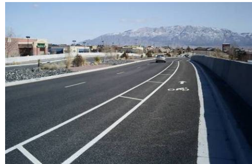
Buffered bike lanes protect cyclists from fast-moving traffic
