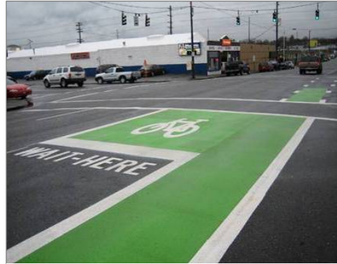
Figure 54. Bike boxes have been installed at several intersections in Portland, OR where right-turning motorists conflict with through bicyclists.
