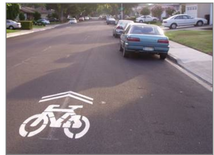
Shared lane markings can be used on minor and major roadways.
