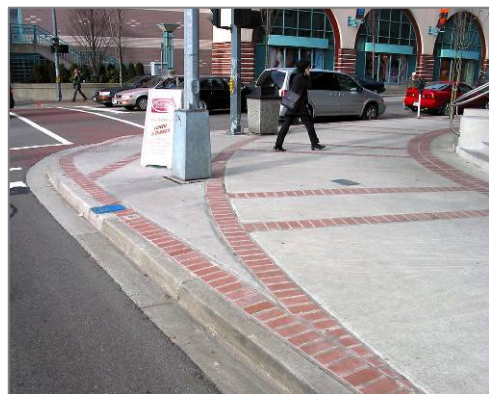
Figure 55. Reducing the radius of a turn reduces traffic speed and greatly improves safety for bicyclists and pedestrians
