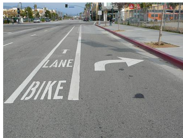
Continuing a bike lane straight while providing a right-turn pocket reduces bicycle/motor vehicle conflicts
