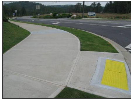
A diagonal curb ramp with detectible warning.
