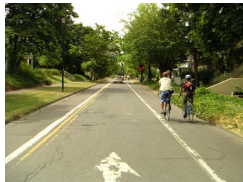
This contraflow bike lane in Portland, OR (left) provides a key connection along a narrow one-way street.
