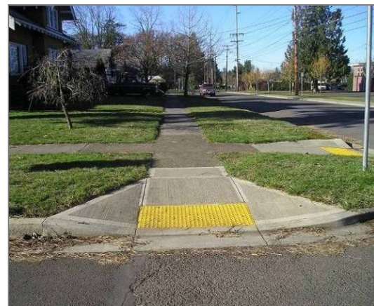
Example of an ADA-compliant perpendicular curb ramp
