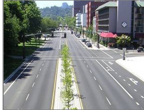
This street previously had 13’ lanes, which were narrowed to accommodate bike lanes without removing a lane.
