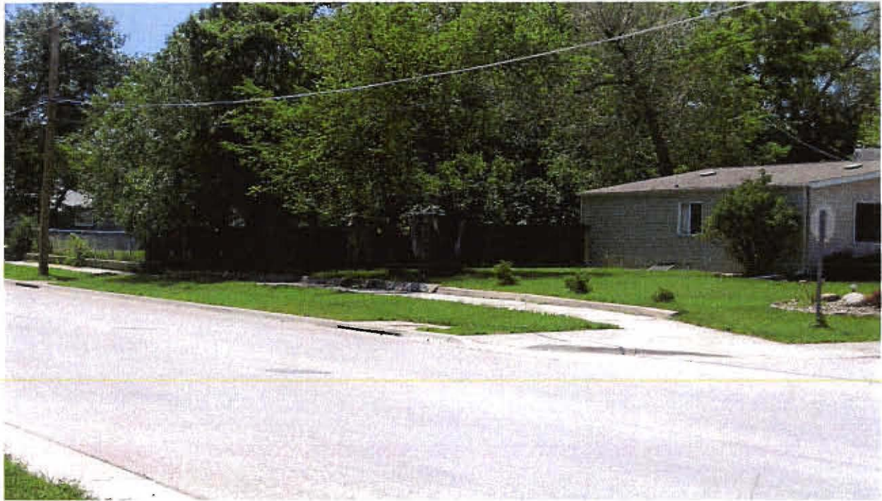
Completed 6 foot fence, corner lot at 713 E. Ohio Street
