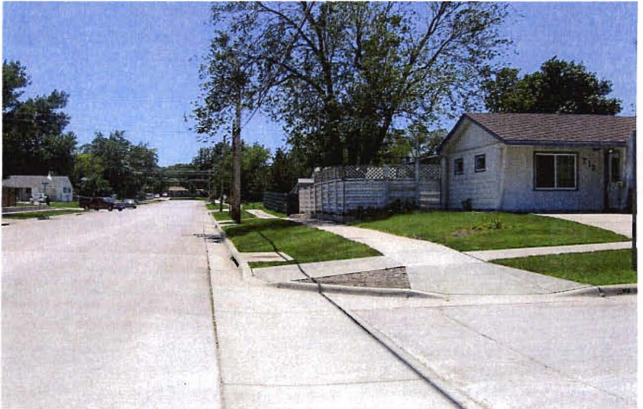
Completed 6 foot fence, corner lot 713 E. Iowa Street
