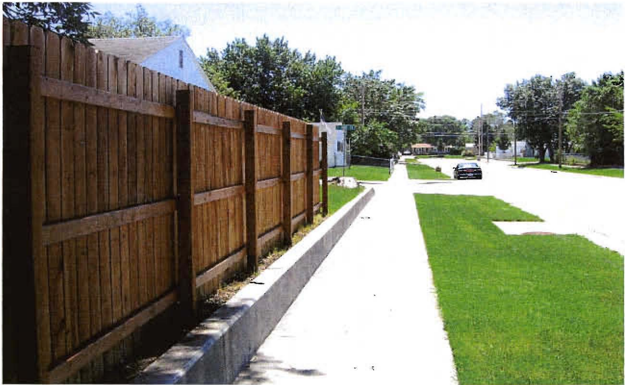
Completed 6 foot fence, corner lot 802 E. Ohio Street
