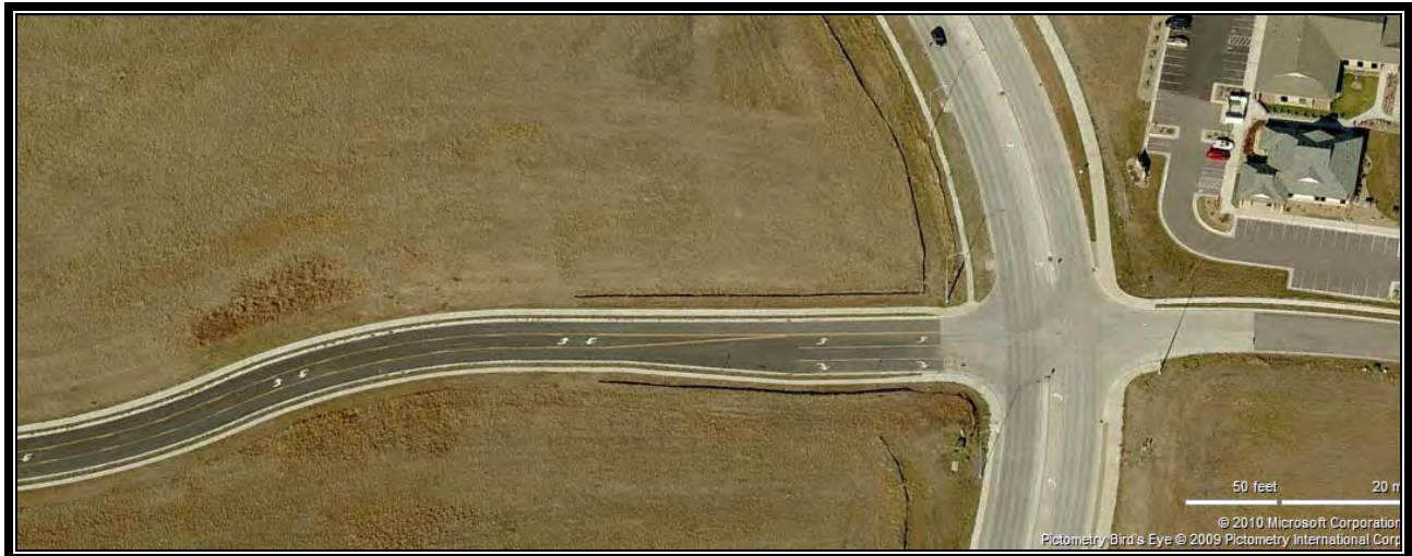
Figure 3: 5 th Street and Stumer Road Intersection
