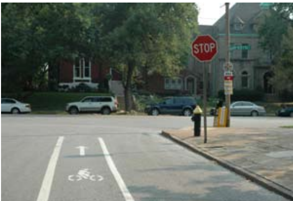
Bicycle boulevards in Berkeley (top) and Saint Louis (above). These streets parallel arterials and provide priority environments for bicycle transportation. Primary investments include removing hazards and providing pavement markings and signage. Bicycle boulevards may use sharrow (shared lane) pavement markings or bike lanes.
