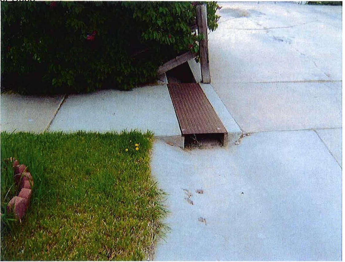
OUTLET STRUCTURE TO HERMAN STREET
