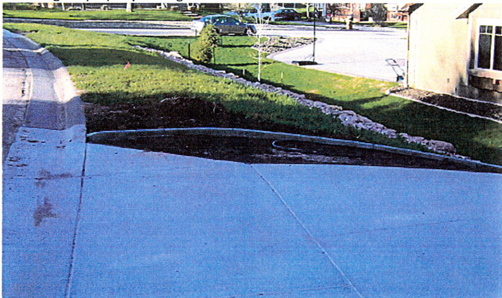
North edge of property looking north.
