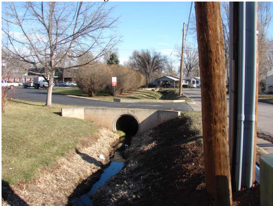
Picture 1. Dover Street Channel along Dover Street
