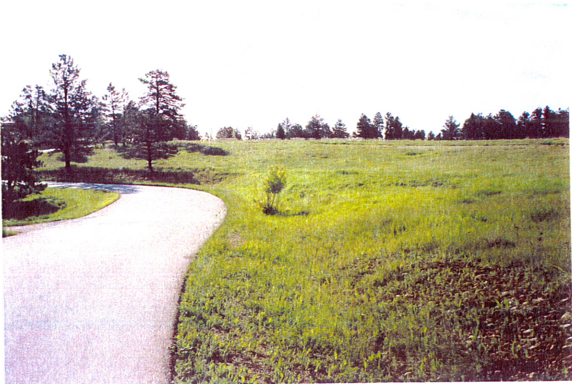
Canterberry Road – south side looking easterly
