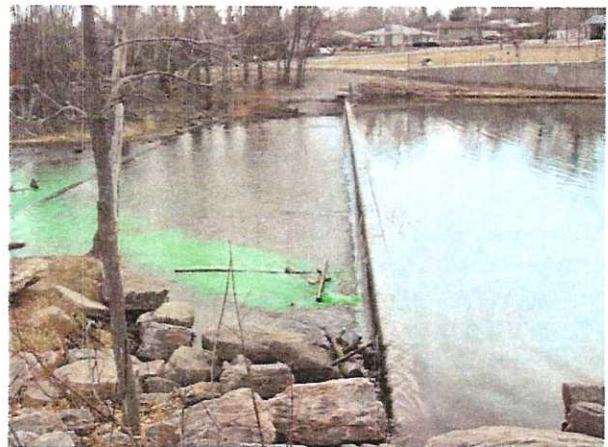
Photos 7 & 8 – March 2005, Midco Diving dye testing shows an extensive amount of dye exiting the underdrain pipe outlet at the base of the concrete apron downstream of the spillway.
