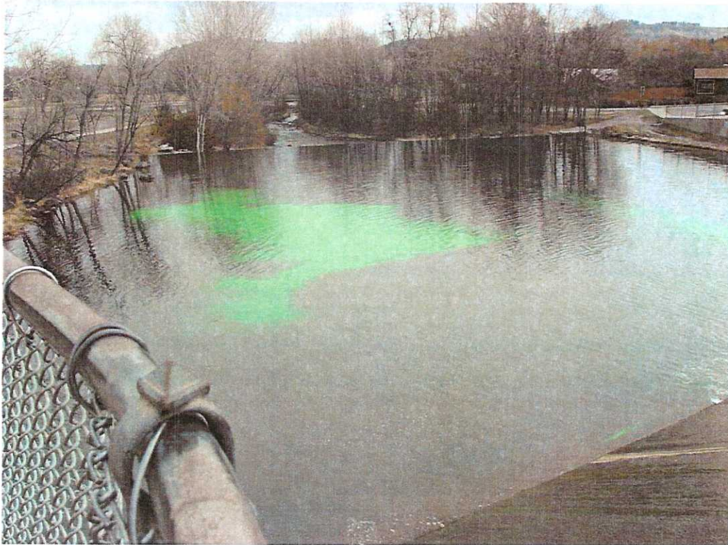
Photo 3 – March 2005, Midco Diving dye testing reveals a dark plume of dye at the area around the existing boil downstream prior to the dye flowing over the spillway.
