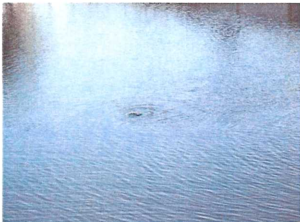
Photos 16 & 17 – Fall 2007, showing the noticeable flow from the seepage boil in the downstream apron.
