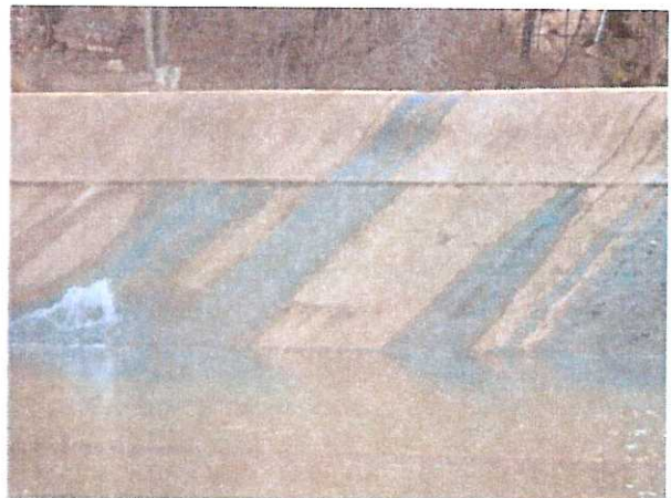
Photos 13 & 14 – Fall 2007, Additional seepage shown by wetted areas around the concrete spillway joints.
