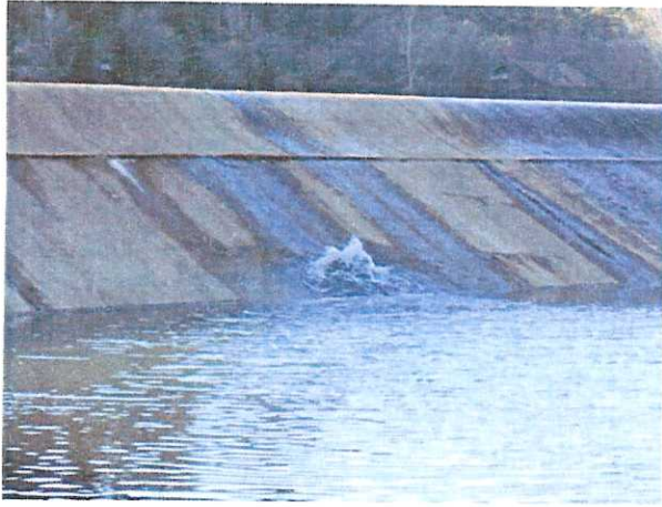
Photos 9 & 10 – Fall 2007, “Roostertail” leak in the concrete face of the spillway.
