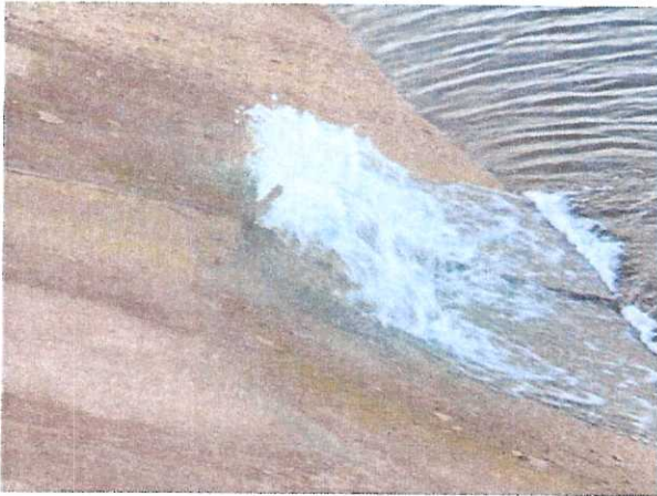
Photos 11 & 12 – Fall 2007, “Roostertail” leak in the concrete face of the spillway.
