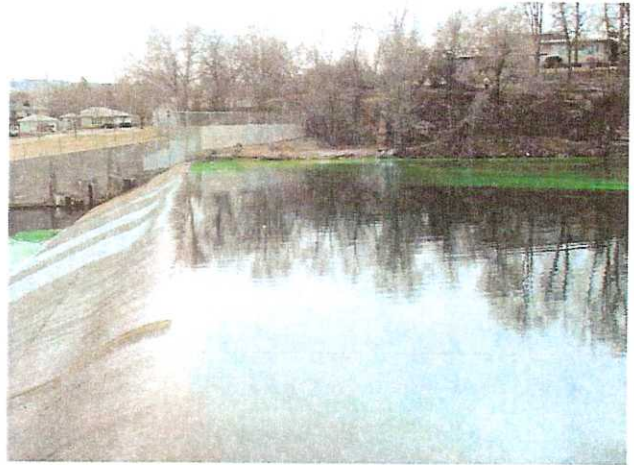
Photos 1 & 2 – March 2005, Midco Diving releasing the dye for seepage testing near the upstream sinkhole.
