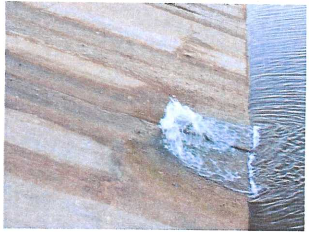
Photos 9 & 10 – Fall 2007, “Roostertail” leak in the concrete face of the spillway.
