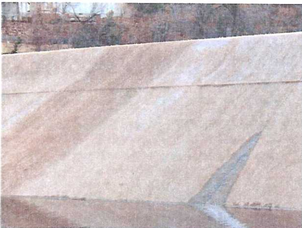
Photos 13 & 14 – Fall 2007, Additional seepage shown by wetted areas around the concrete spillway joints.
