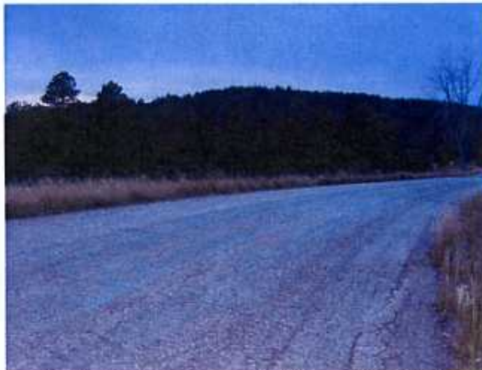
Figure 3 - Chuck Lien Driveway – 1994 Completion (Driving Surface)
