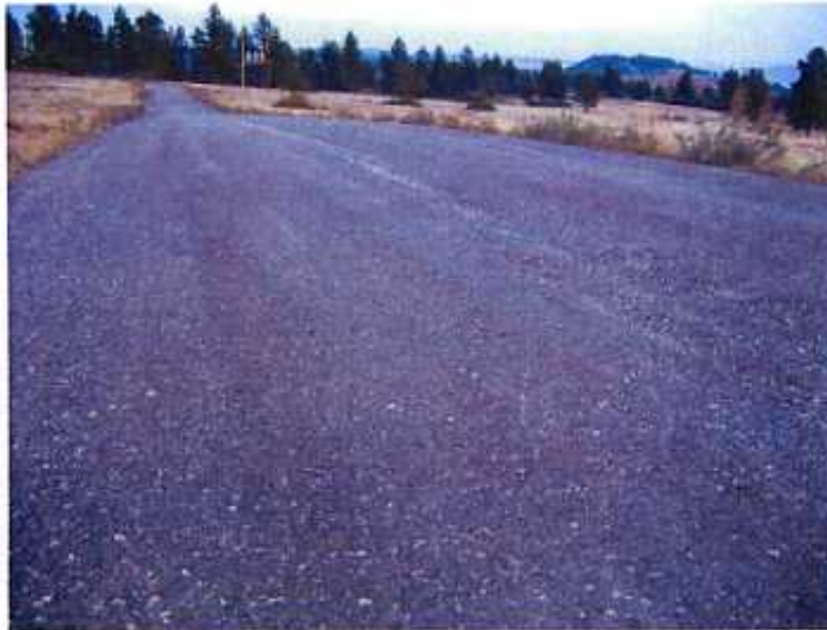
Figure 9 - Pete Lien Driveway – 2005 Completion Date (Driving Surface)
