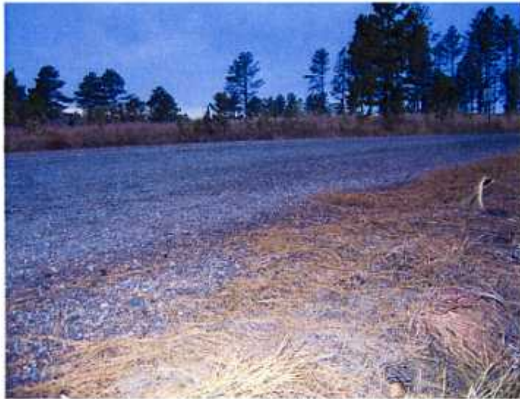
Figure 5 - Bruce Lien Driveway – 1994 Completion (3-4" Thickness)
