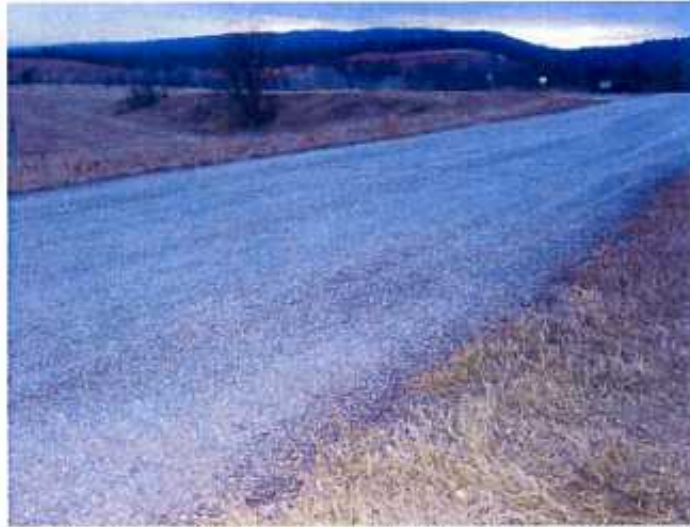
Figure 2 - Chuck Lien Driveway – 1994 Completion (3-4" Thickness)
