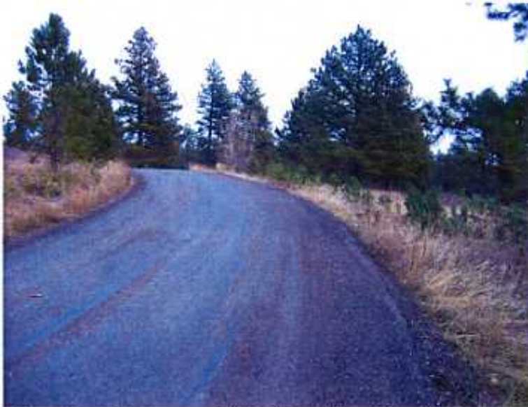
Figure 7 - Pete Lien Driveway – 2005 Completion Date (Current Appearance)
