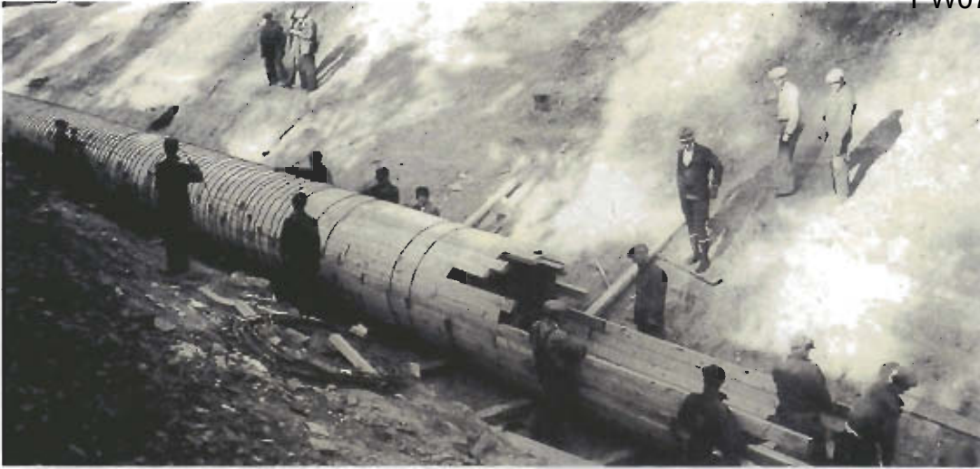
The flume that fed water to the Big Bend Power Plant was built by hand using hundreds of laborers.
