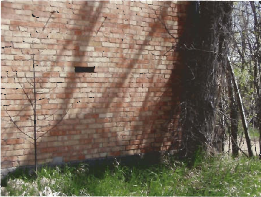
TREE AT SOUTHWEST CORNER
