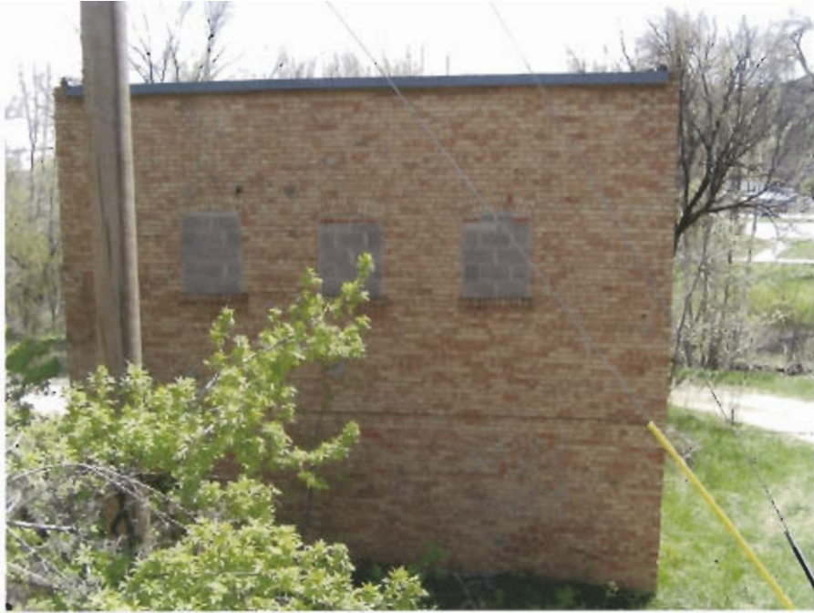
VIEW FROM NORTH
