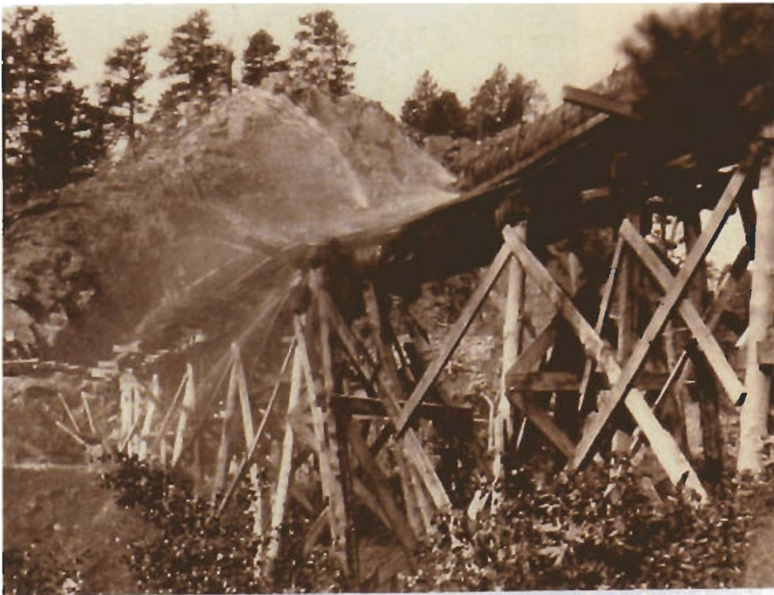
Repairing leaks in the flume was an ongoing job.
