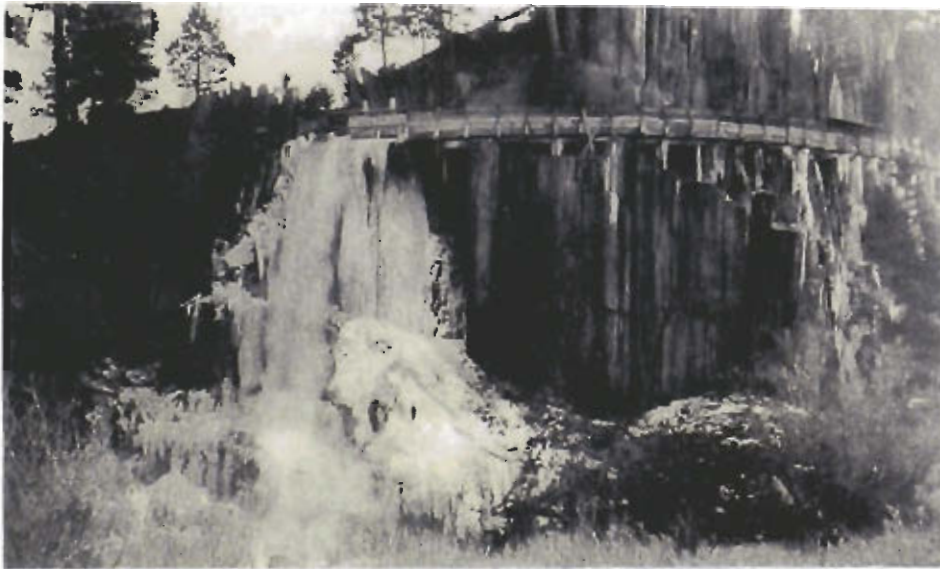
On very cold days the Big Bend Power Plant would shut down because of the frost build-up in the flume.
