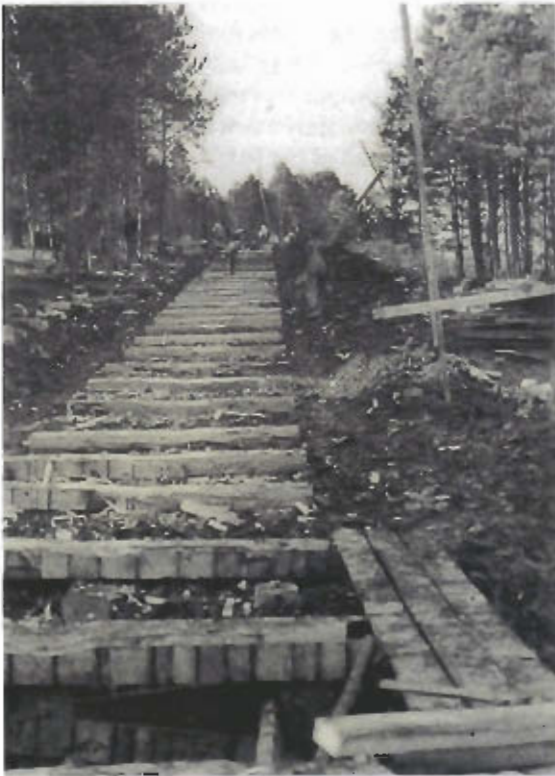
Workers laid the foundation before installing the flume.
