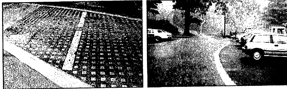
Left: Fig. 20: Belgium block pavers in parking bays (Photo Credit: The Low Impact Development Center)
